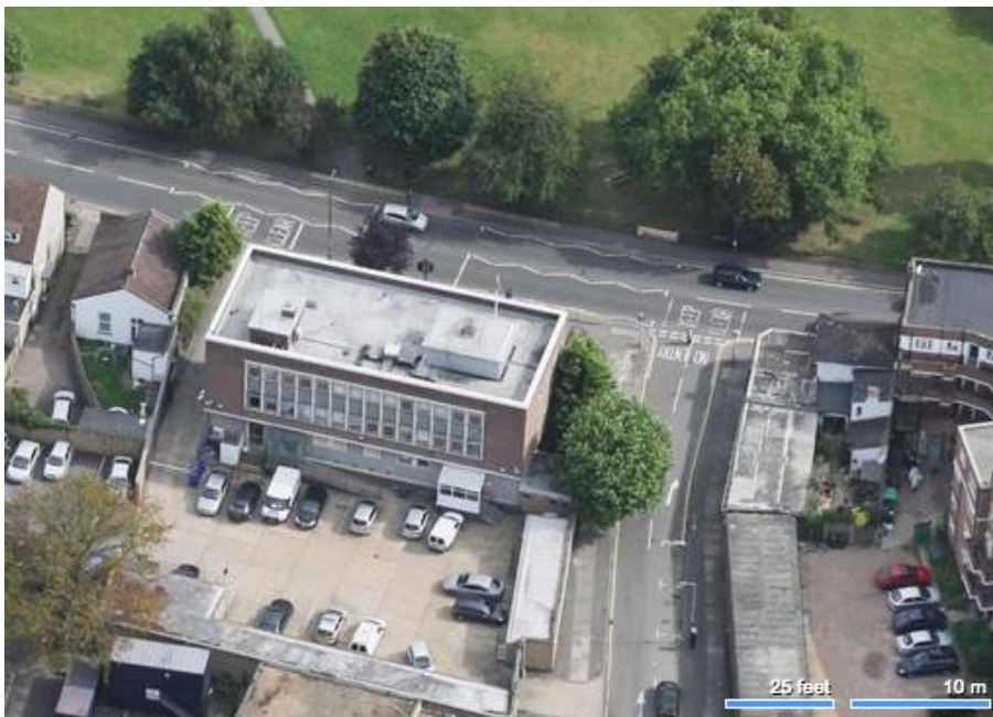
Mitcham Police Station - rear
