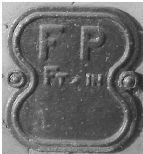
'F P' meant 'Fire Plug', an older name for a fire hydrant. The distance from the plaque to the hydrant is shown underneath in feet, and the size of the water pipe in inches.
