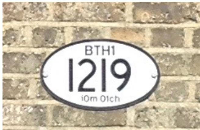
'BTH1' is the Engineer's Line Reference, which identifies the section of track, which is *South Bermondsey Junction to Sutton (East) Junction*, with the terminus being London Bridge station. The number 1219 identifies this bridge.
